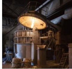
Oxy-Fuel Burner at Ladle Pre-reheating
