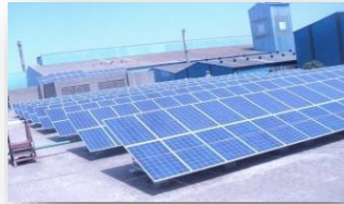
Addition of 4.8 MWP roof-top solar plant
