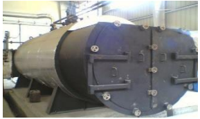
Steam generation by Waste-heat recovery-HBA
